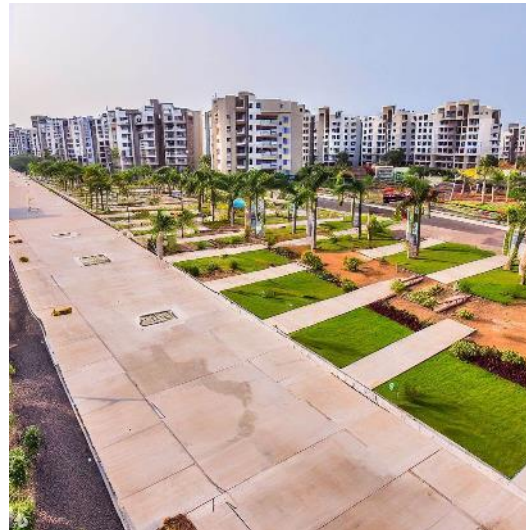
Roads and compound walls
