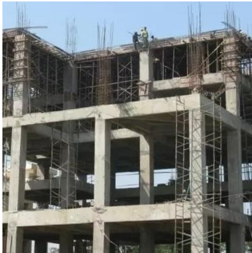
Foundations and structures
